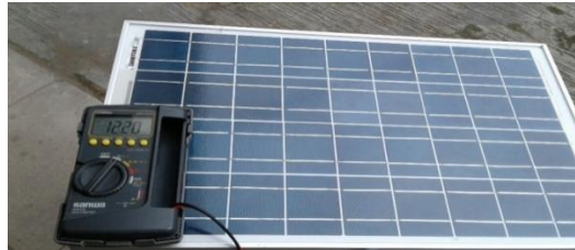
Gambar 4.2 Proses pengukuran tegangan panel surya
