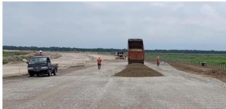
Gambar 1: Alat berat dump truck (Jalan Tol Binjai Langsa, 2021)
